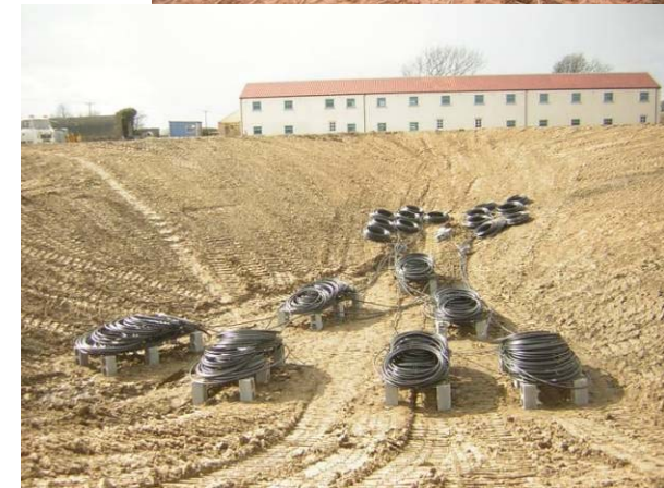
Water source heat pump
