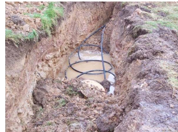
Installing ground loops
