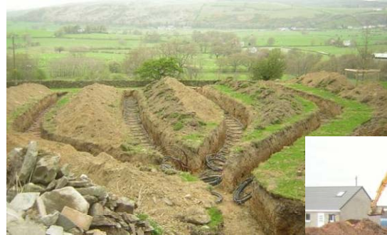
Linear ground pipes
