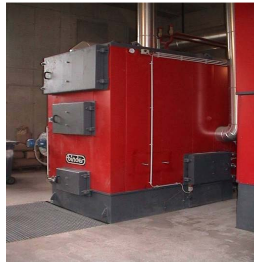
Wood chip boiler
