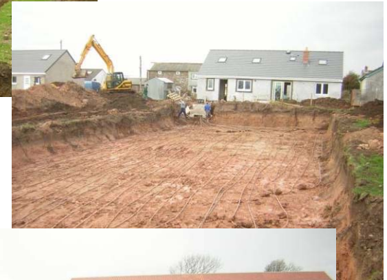
Linear ground pipes
