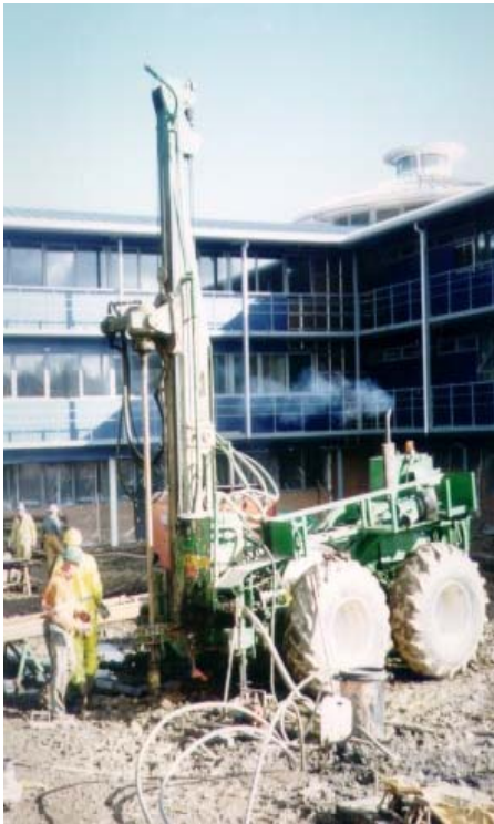
Drilling a borehole
